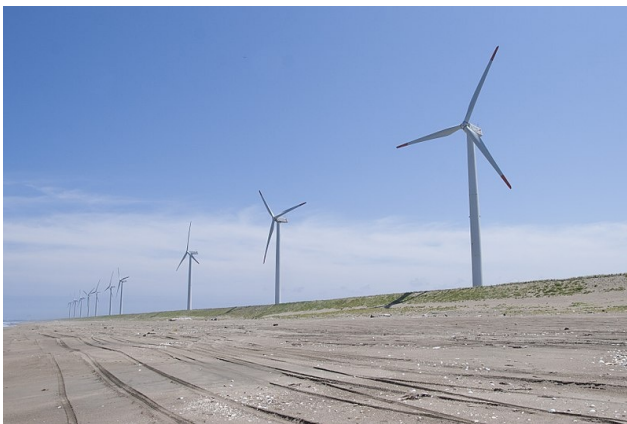
Hasaki Wind Farm
